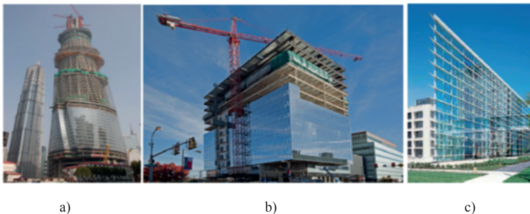
Fig. 6. Construction of curtain walls, architectural systems broadly utilise the principles of modular design, manufacture and on-site assembly: a) Shanghai Tower Curtain Wall (China), b) Science Research Centre, Wausau (Pennsylvania/US), c) Stick System curtain wall Reliance™ manufactured by Oldcastle [11].
