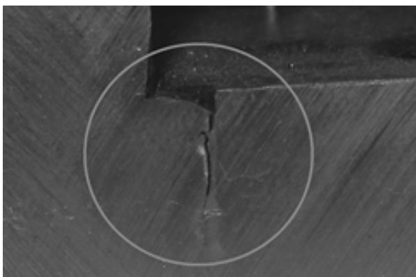
Fig. 15. Cracks in the device frame
